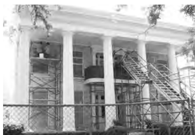
Fencing and balcony protection.
