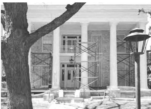
Scaffolding is installed for conservation of columns.
