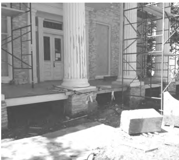
Scaffolding is installed for conservation of columns.
