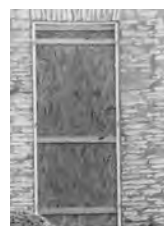
Windows were boarded up and interior floors were covered.
