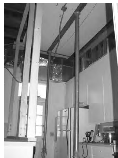
Construction in kitchen.
