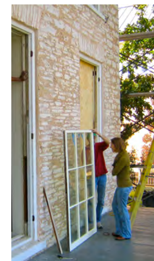
Rowena Dasch and a master carpenter inspect a window sash.
