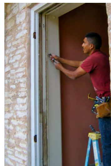
Window with the sash removed. Multiple coats of paint and built-up finish were removed to restore the window to its original condition.
