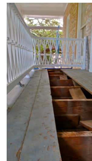
Inside the balcony support system.
